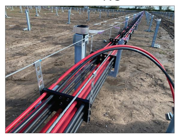
Solar Snake Max XL conveyance accommodates cables ranging from 350 Kcmil up to 750 Kcmil within one universal click support module. The easy snap together components are designed to maintain NEC 310.15 code compliant cable separation with no requirement to derate the cables. This patented trenchless solution substantially decreases construction cycle times and material costs.
