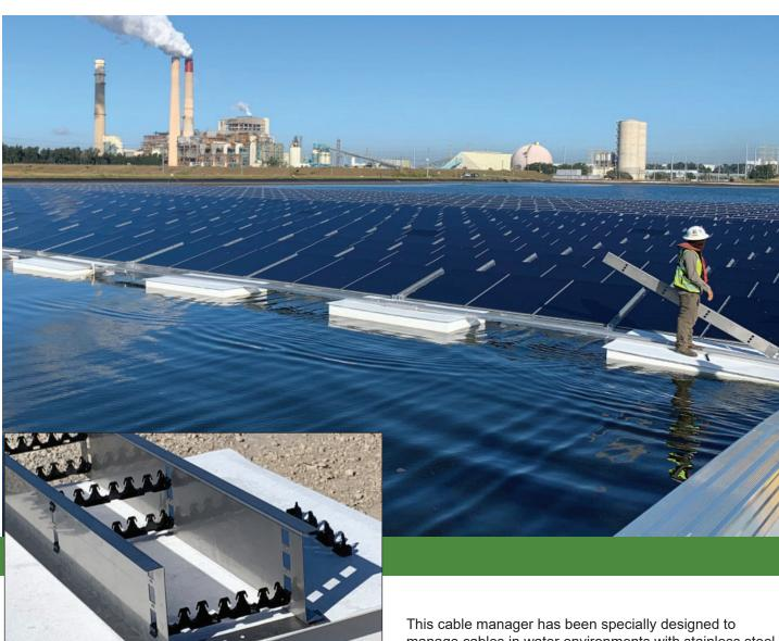
This cable manager has been specially designed to manage cables in water environments with stainless steel rails and snap together Solar Snake Max clicks to maintain NEC 310.15 code compliant cable separation.
