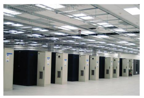
Snake Tray's Mega Snake is deployed in this data center. The system offers several egress methods from either the side of the tray or along the tray's bottom. It also offers several types of reducing transitions that can be used to reduce tray sizes.
