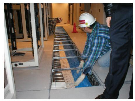
Snake Canyon is a 2-by-2-foot modular tray solution for the raised floor environment that can be deployed at multiple elevations under the floor. It fits within the floor's grid pattern.
