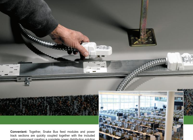
convenient: Together, Snake Bus feed modules and power track sections are quickly coupled together with the included splice component creating a complete power distribution solution for the raised floor environment. Individual power modules are then attached to the Snake Bus track system making installation and retrofits simple and easy for both large and small scale installations.
