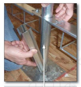
Install riser tube onto existing pedestal by snapping the tube over the pedestal and adjust to the correct height. Note: The Latch LOC basket will sit on top of the riser not the adjuster nut as shown in the photo below.
