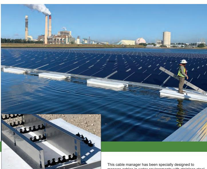
This cable manager has been specially designed to manage cables in water environments with stainless steel rails and snap together polycarbonate clicks to maintain NEC 310.15 code compliant cable separation.
