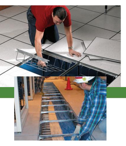
Snake Canyon has revolutionized the way cables can be installed in computer access floors. This modular cable tray system instantly integrates with the existing structural elements of an access floor to create the fastest way to install under-floor cable tray.
