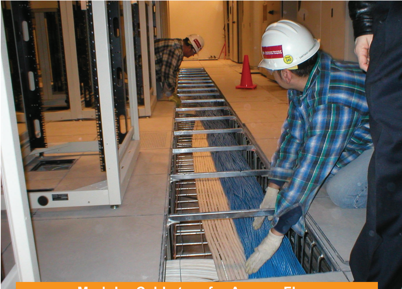
Modular Cable tray for Access Floors
