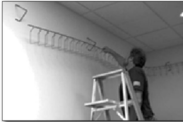
Figure 4 - Installing Snake Tray on a wall using WBN wall brackets.
