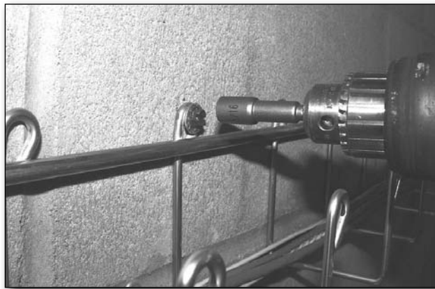
Figure 6 - Wall Snake attached directly to the wall using CM-501-CA anchor bolts
