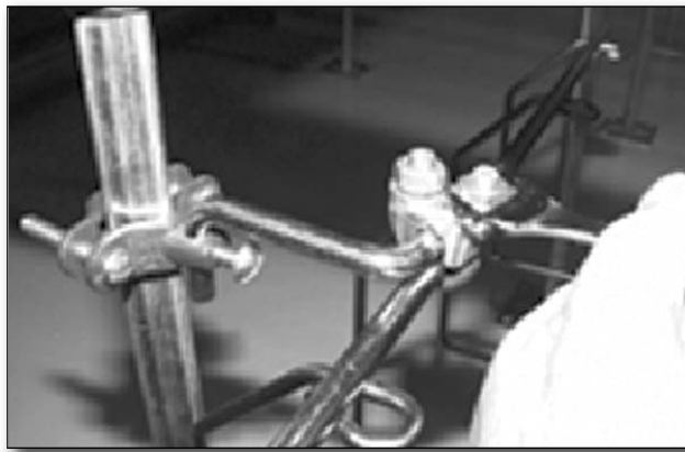
Figure 5 - Securing the 201 Series Snake Tray under an access floor to the vertical pedestal base using the ST-201 bracket.
